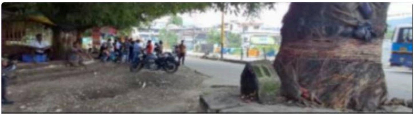
Vertical height clearance and bad condition of the road
